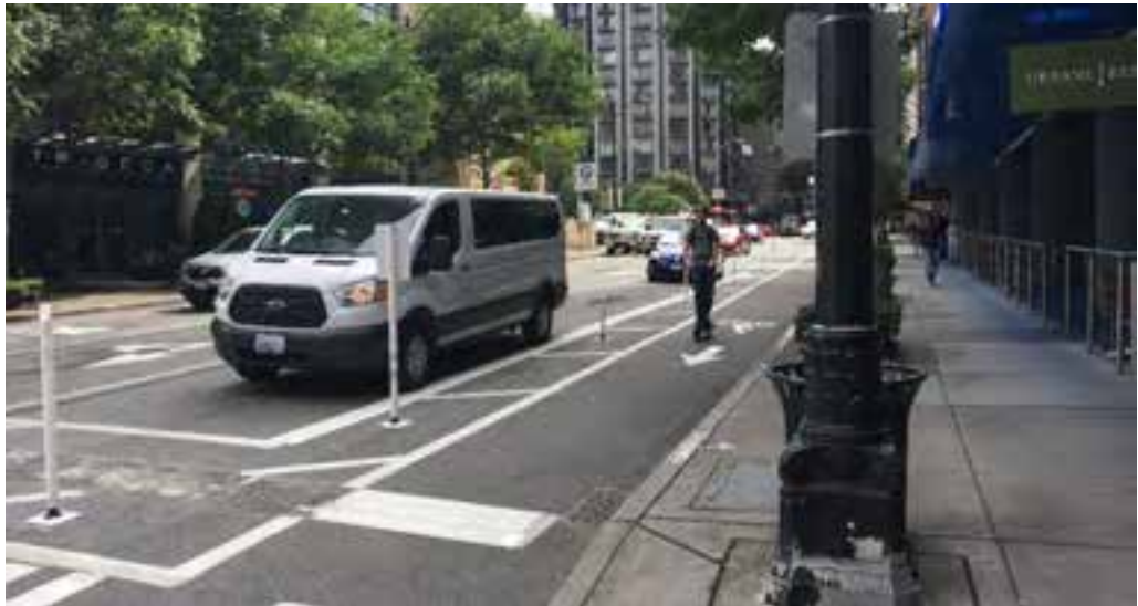
One-way Protected Bike Lane with Delineator Posts
