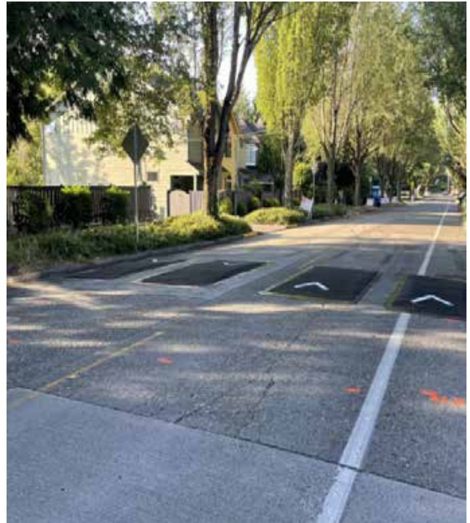
Speed cushions on 15th Ave S between Atlantic & Massachusetts help to slow traffic.
