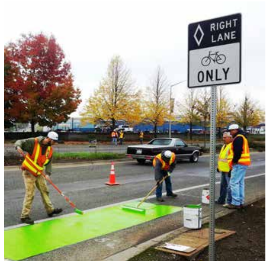
Crews painting a green bicycle lane
