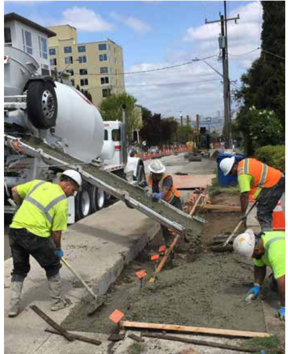
Construction crew at work in West Seattle
