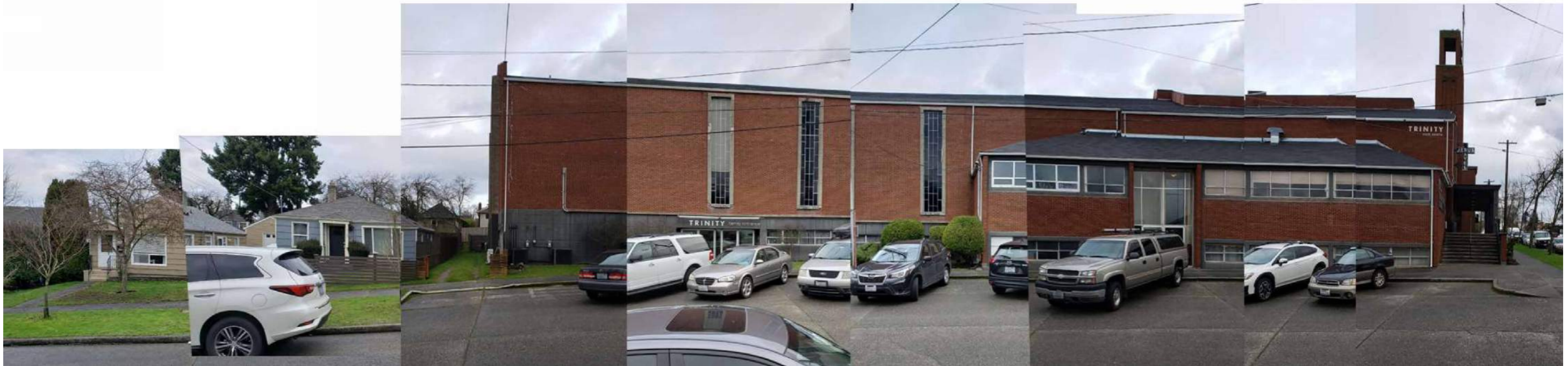
SW IDA ST LOOKING NORTH
