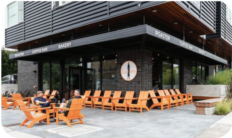
outdoor dining provides break in street wall
