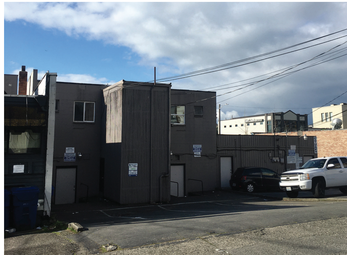
4 View west from alley
