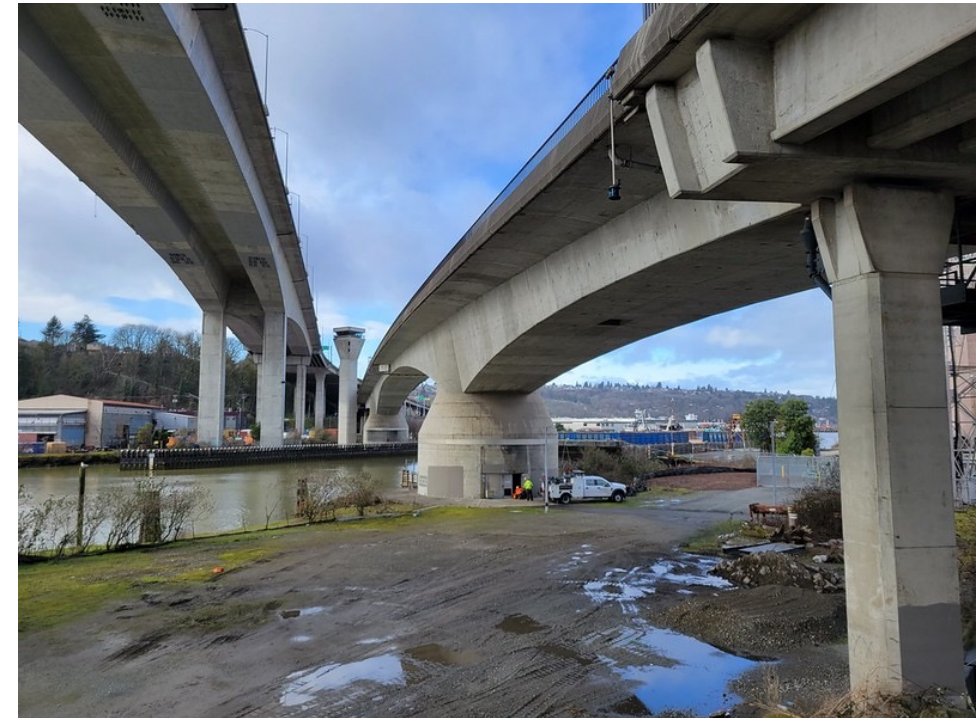
The control tower for the Spokane St Swing Bridge (low bridge) is nested between the low and high bridges
