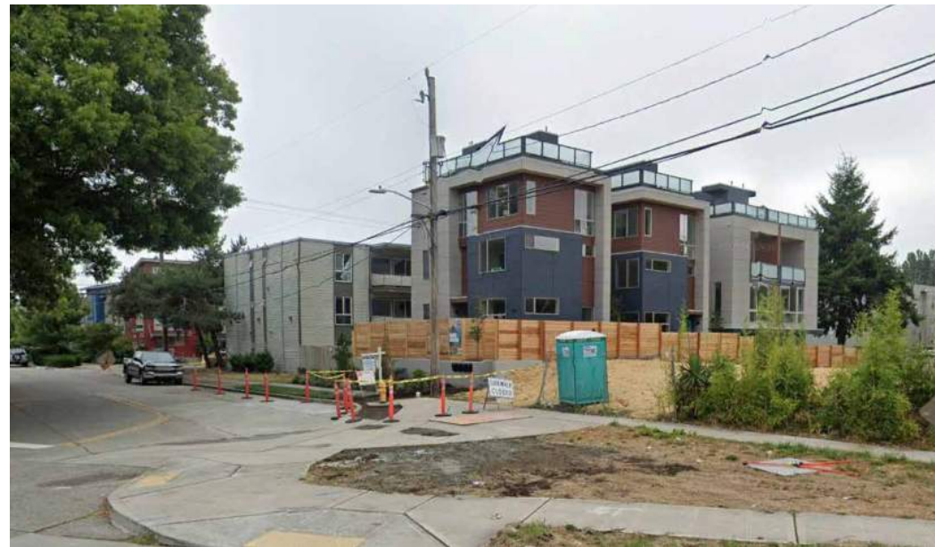
1 LOOKING NORTH ON 18TH AVE SW
