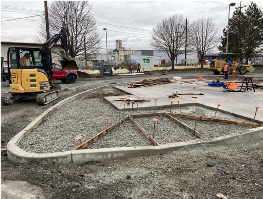
ADA Ramp outside admin building
