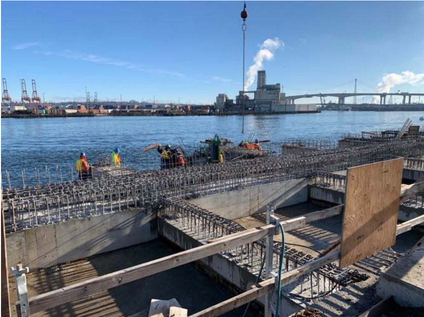
First section dock asphalt
