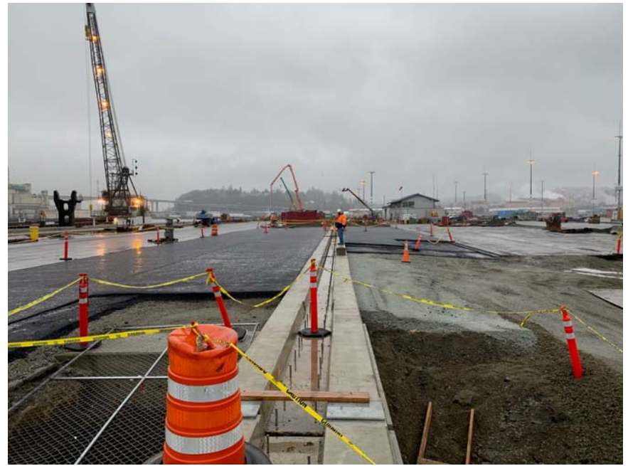
Asphalt at LSCR
