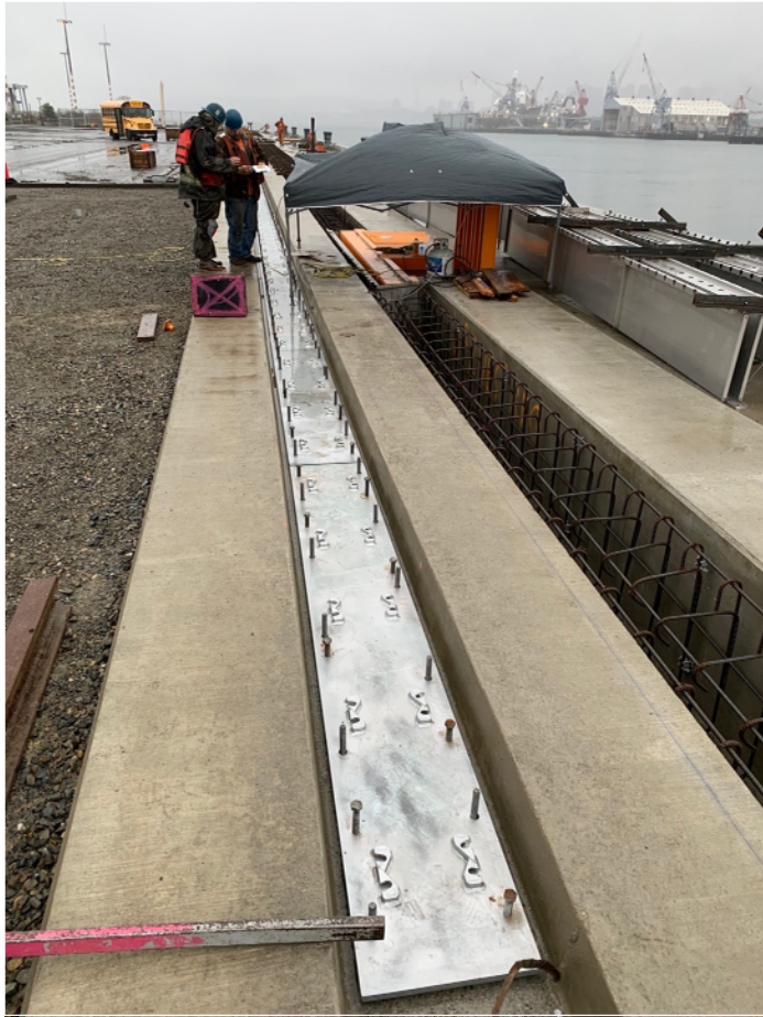
Crane Rail Hardware
