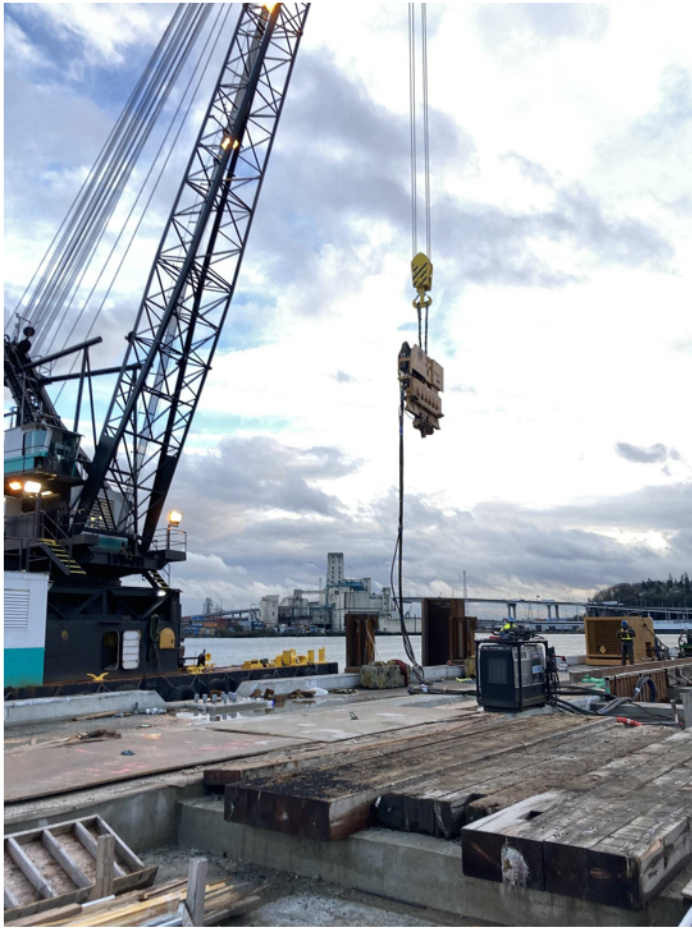
Hammer for the toe wall pile
