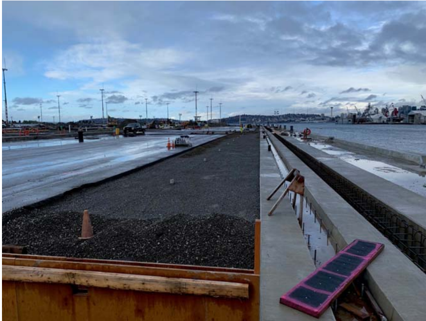
Backfill area between WSCR and asphalt
