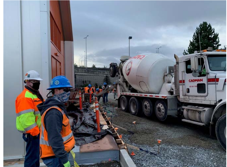
Pouring curb at substation
