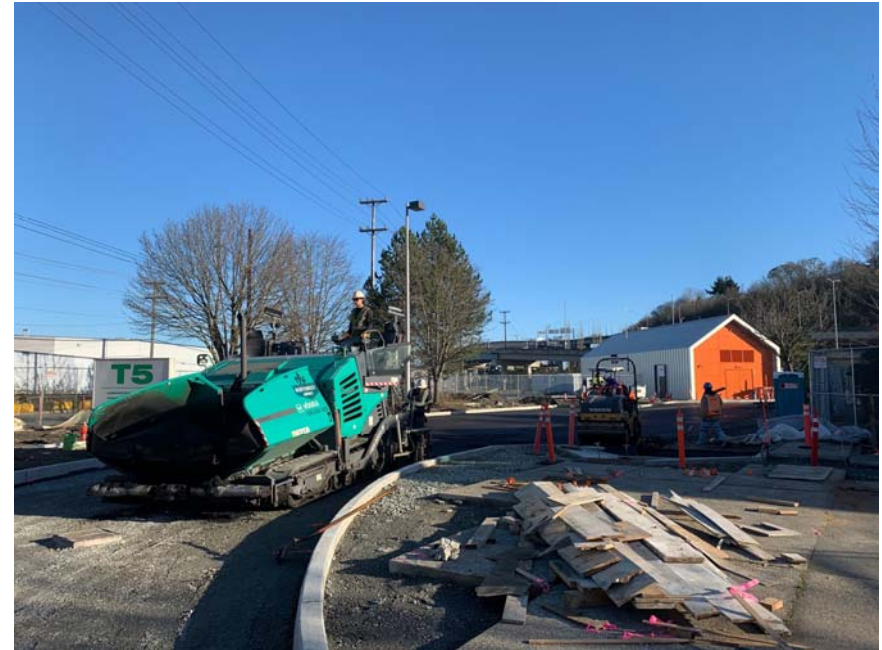
Paving at substation
