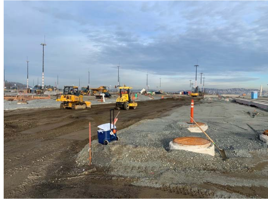
Paving prep at north end
