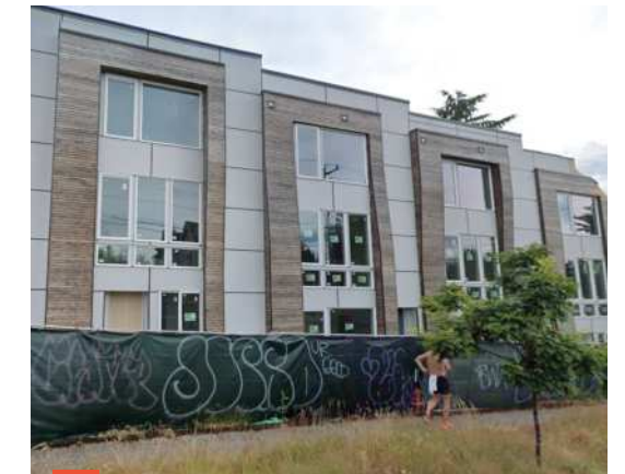
3 new townhome construction
