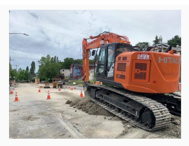
As part of this project, we will be upgrading the roadway throughout the corridor. The roadway above has been fully demolished and is getting prepared for paving. Driveways will be closed as we repave the roadway. You can expect roadway demolition to look like the photo above.
