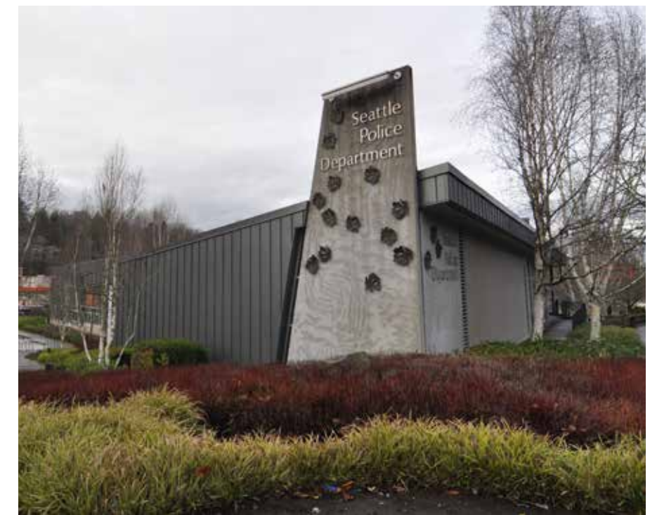
9 SW Precinct Police Station 2300 SW Webster St Built: 2002
