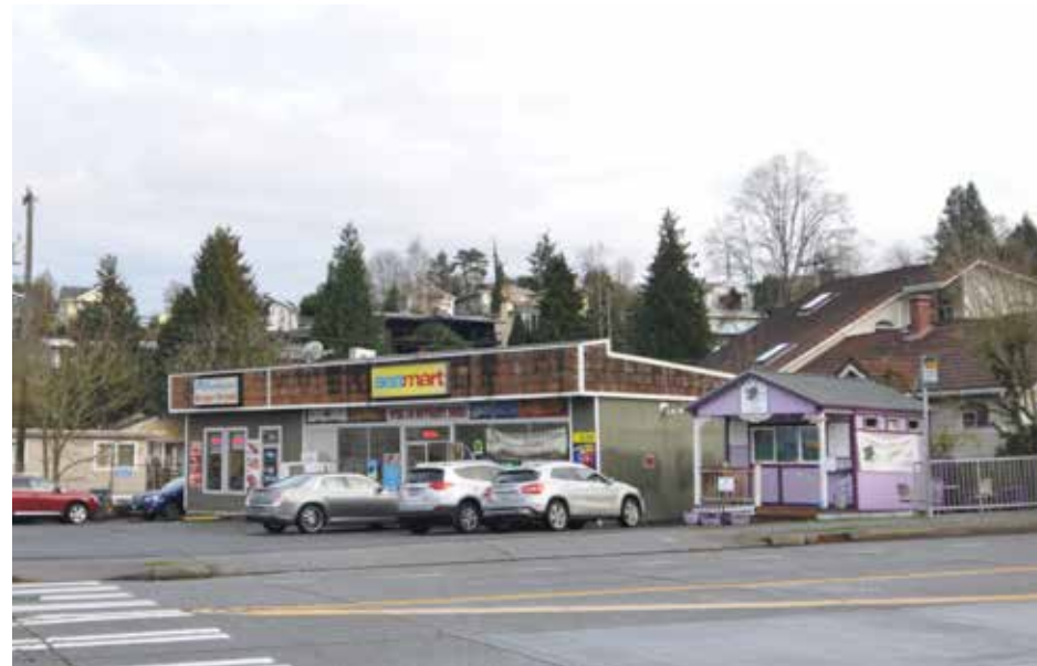
④ Commercial storefronts along SW Holden St
