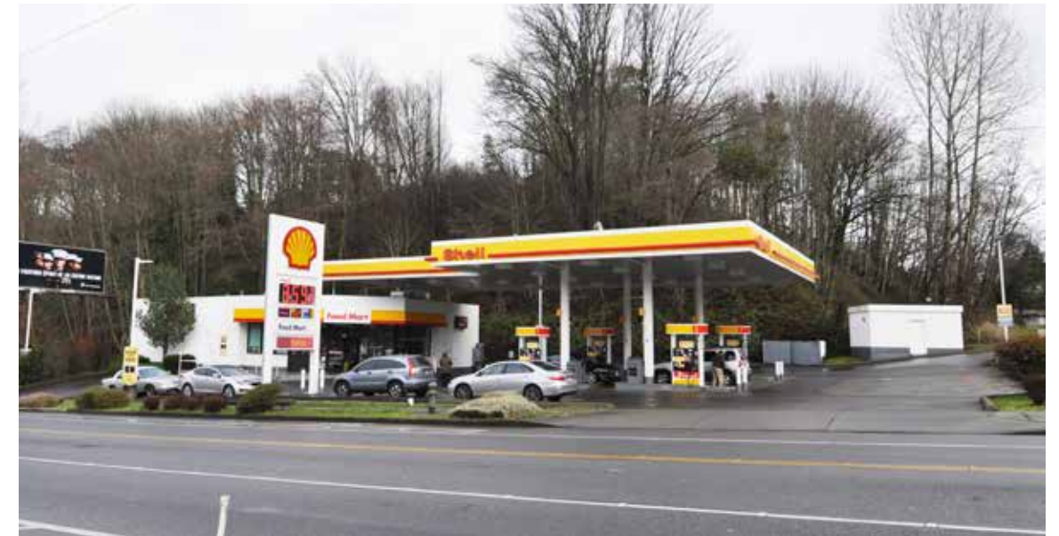
1 Convenience Store with Gas along Delridge Way SW
