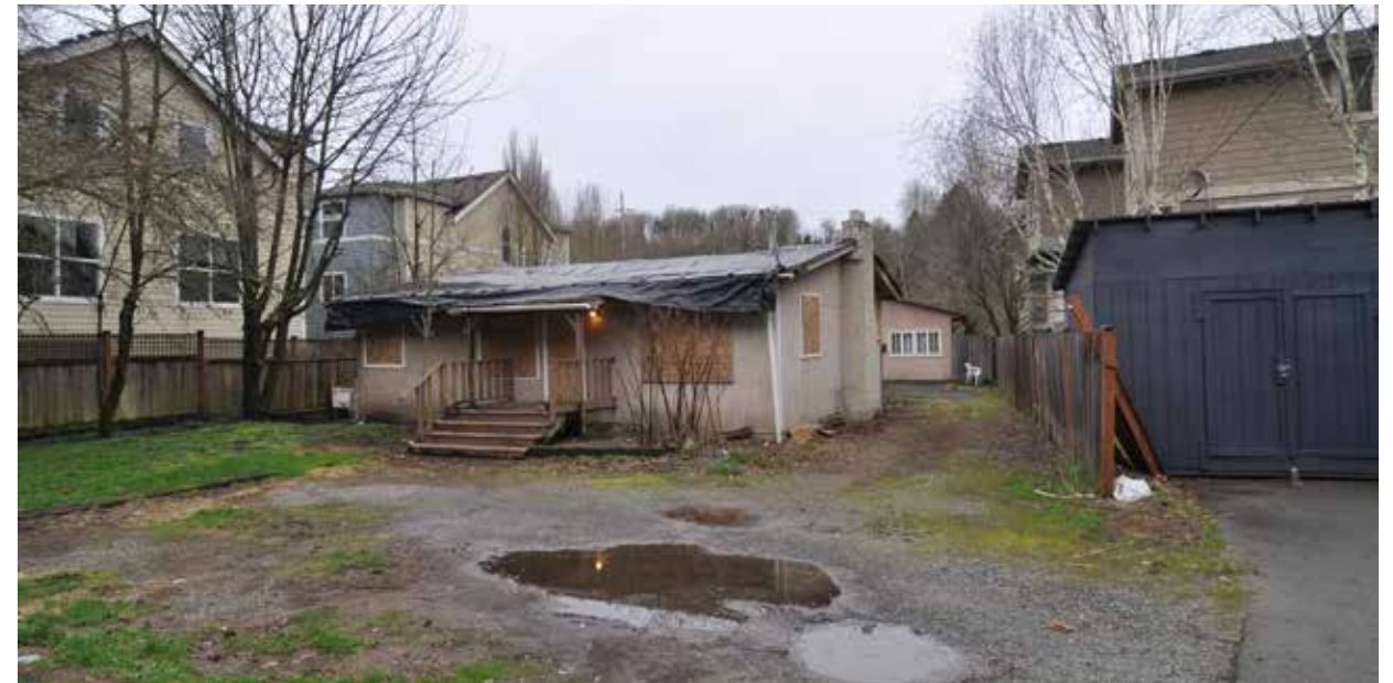
① View facing Southwest looking at site
