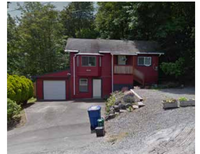
⑫ Single Family Residence 2431 SW Myrtle St Built: 1942
