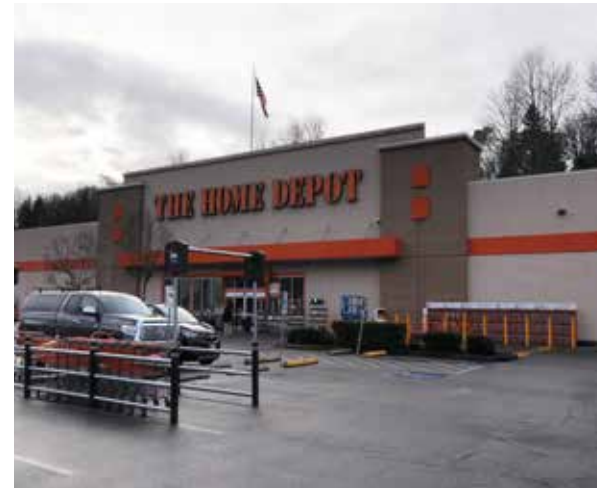
③ Home Depot 7345 Delridge Way SW Built: 2005
