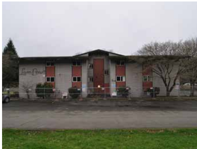
⑨ Lam Bow Apartments 6935 Delridge Way SW
