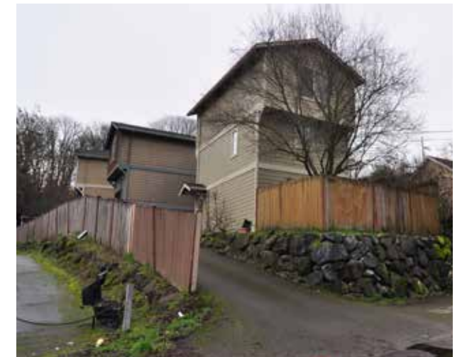
④ Townhouses 6966 23rd Ave SW Built: 2005
