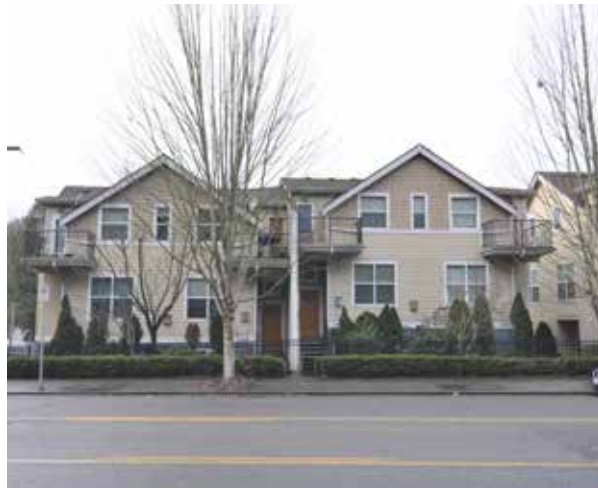
④ Townhouse Development 2202 SW Myrtle St Built: 2006, 14 Units
