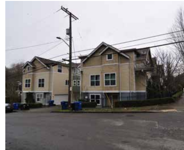
① Townhouse Development 2202 SW Myrtle St Built: 2006, 14 Units
