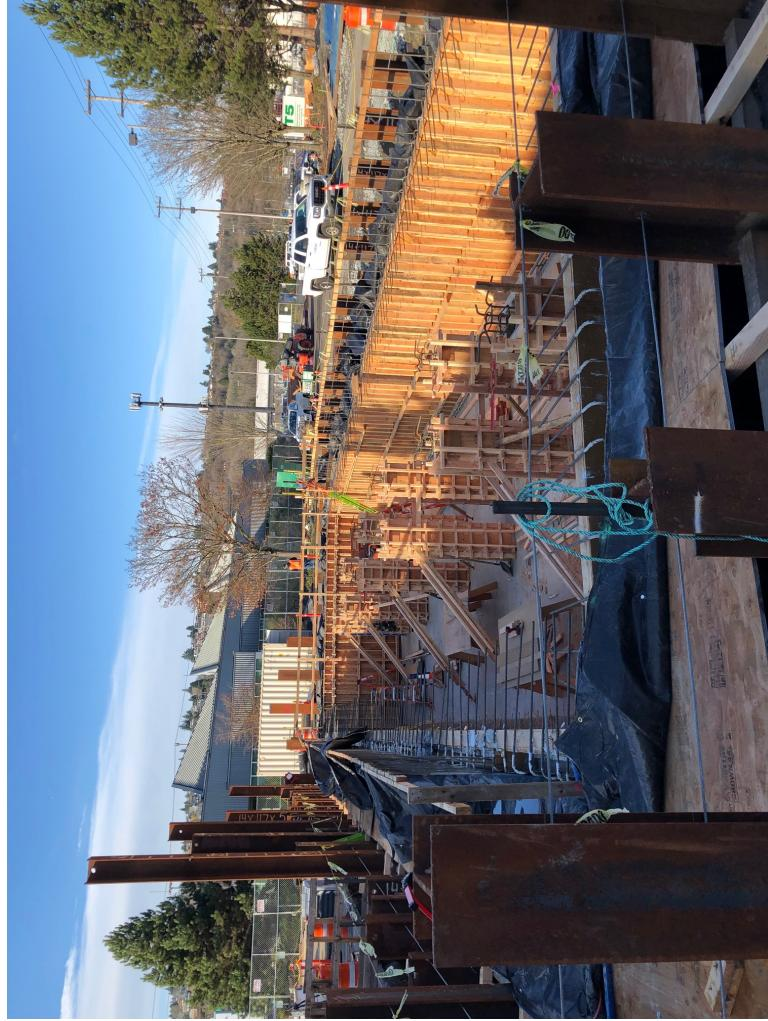
*Construction continues on the new Terminal 5 primary substation that will provide increased power to include shore power capabilities.*
