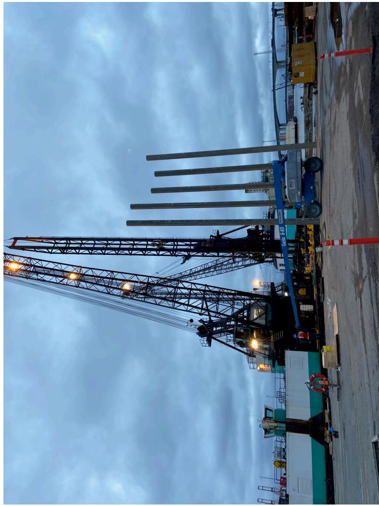
*A temporary over-water structure (falsework) is being installed at Terminal 5 that will support the new cast-in-place concrete wharf structure while the concrete is curing.*
