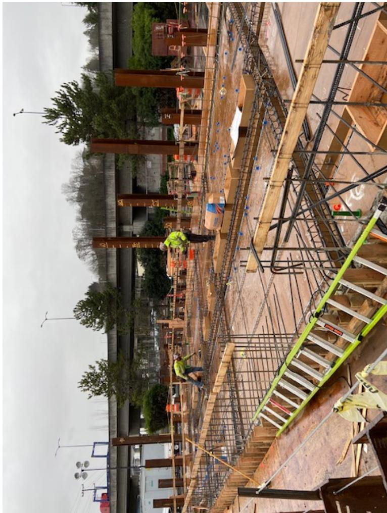
*Crews removed piles and pile caps to make way for upgraded beams, piles, and deck panels. These dock upgrades will support the weight of larger cranes.*
