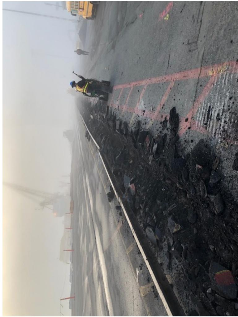
*Piles are being driven through trenches and a concrete beam will be placed on top of the piles to strengthen the foundation for the new landside crane rail beam.*
