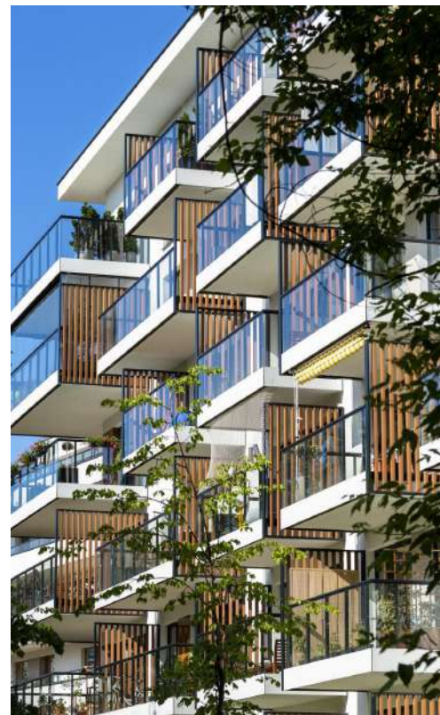
secondary architectural features
