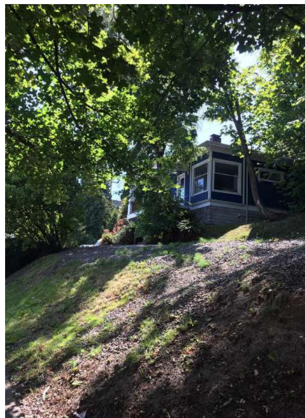
3 view up to site from Harbor Ave
