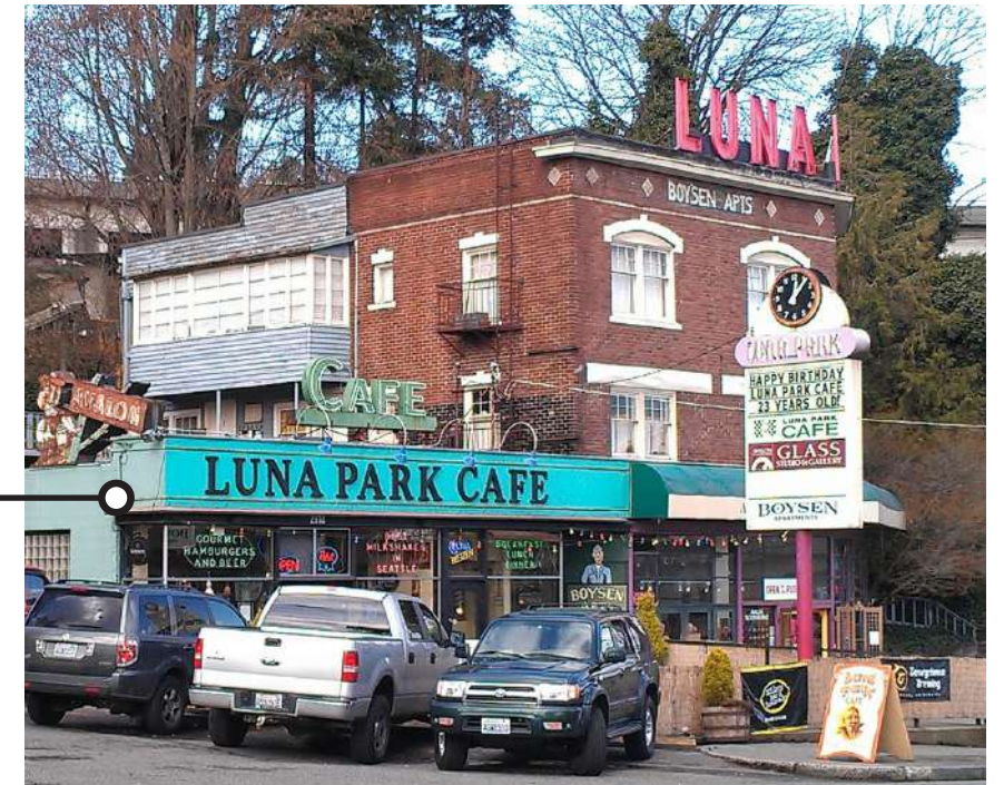
material separation at base
