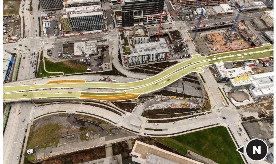
North SR 99 tunnel portal
