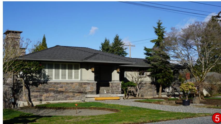
Two Part Composition Facade; Window Facing View
