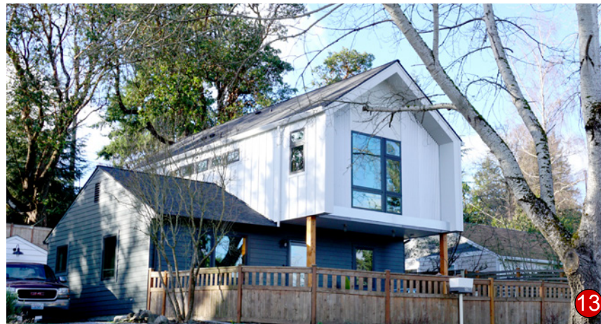
Window Facing View; Board and Batten Facade; Decks; Tongue & Groove Wood; Top & Bottom Composition
