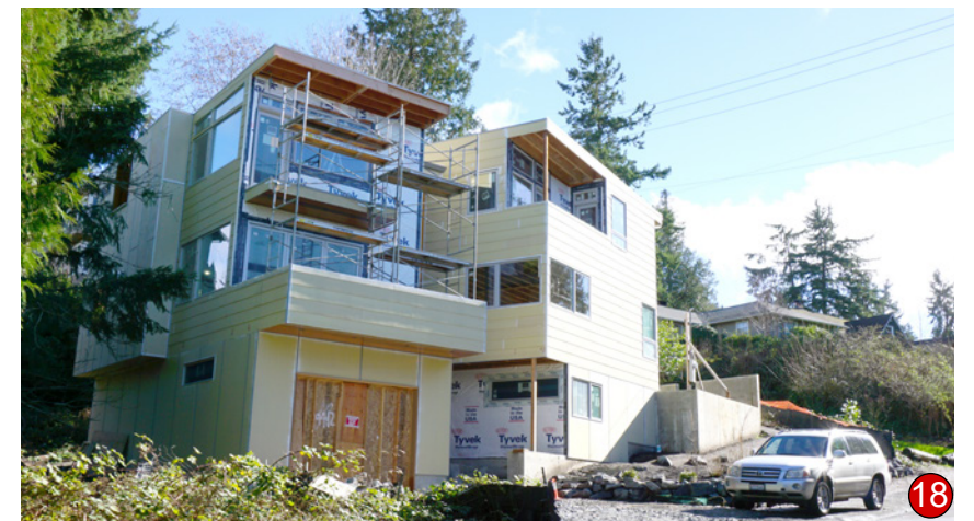
Large Windows Facing View; Roof; Decks;
