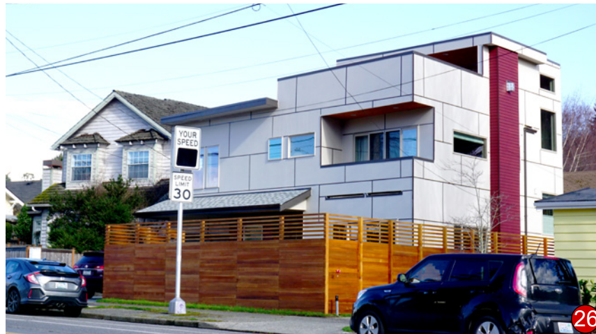
Fiber Cement Cladding; Decks; Roof; Penthouse 26
