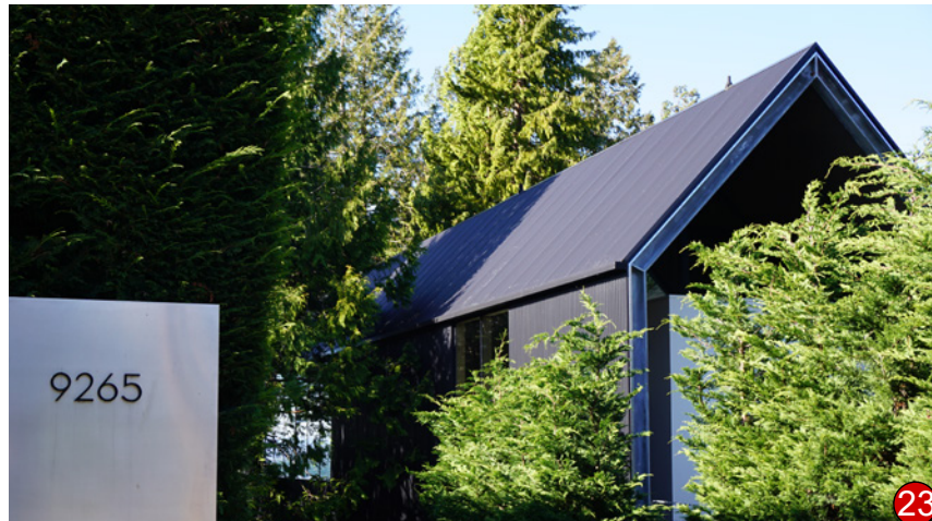
Roof; Metal Cladding 23
