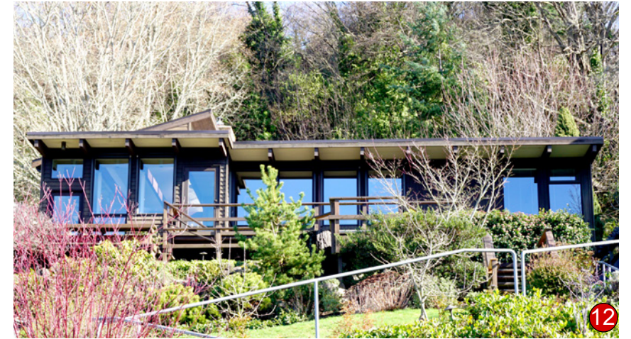
Roof; Decks; Large Windows Facing View; Wood Cladding
