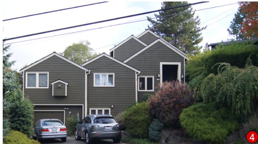
Windows Facing View; Undulating Roof
