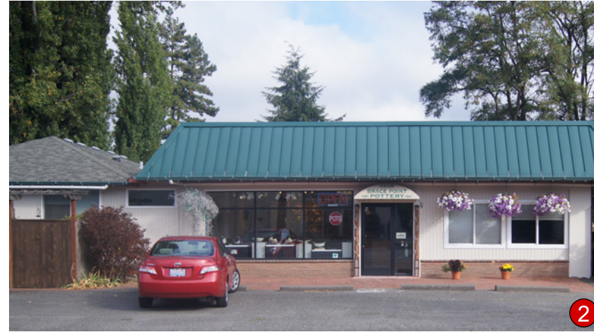
Building Adjacent to Site
