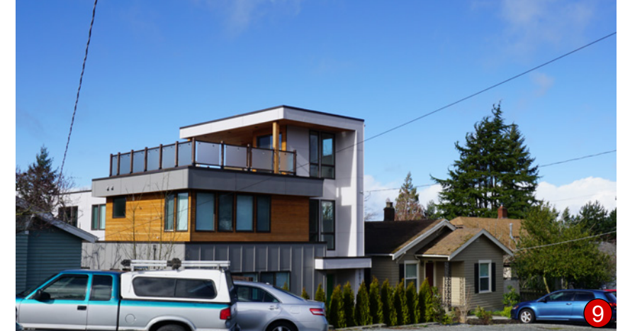
Roof; Wood Cladding; Fiber Cement Cladding; Window Facing View; Metal and Glass Railings; Landscape along Street
