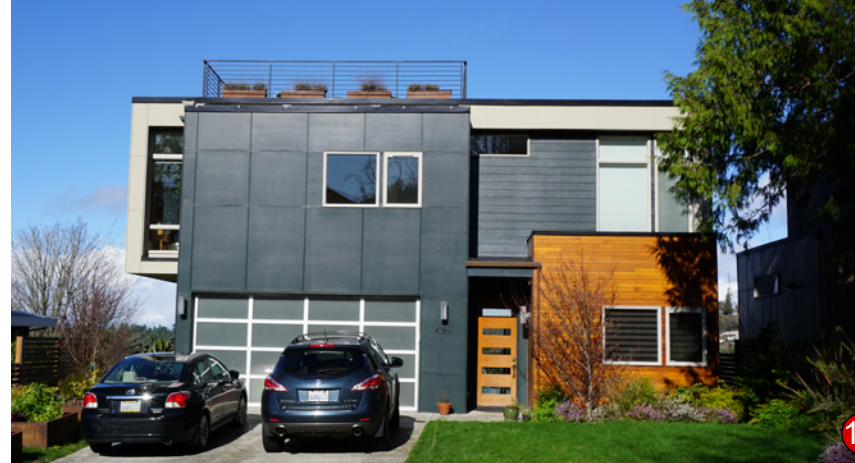
Roof; Deck; Fiber Cement Cladding; Wood Cladding
