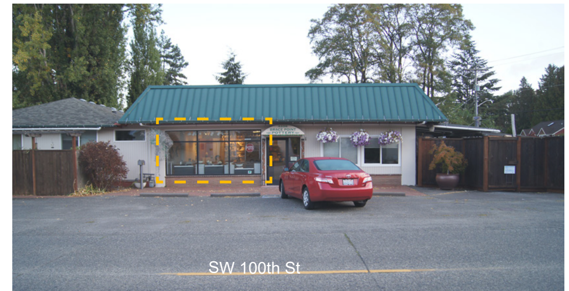
Brace Point Pottery Storefront
