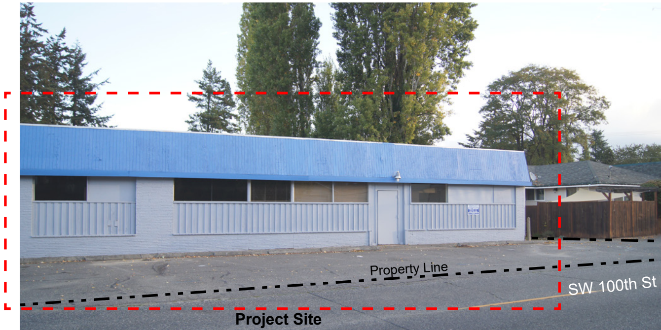
Existing Structure on the Project Site
