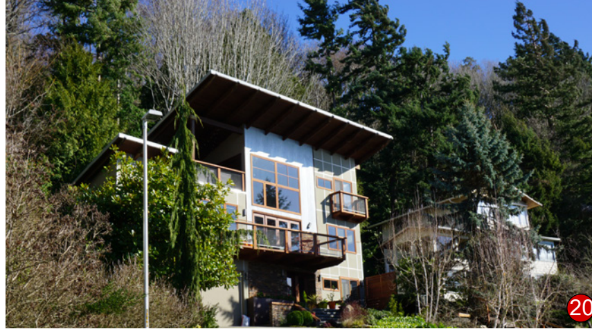
Roof; Decks; Fiber Cement Cladding; Metal Cladding 20
