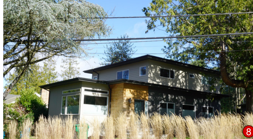
Wood Entry; Fiber Cement Cladding; Roof; Window Facing View; Landscape along Street
