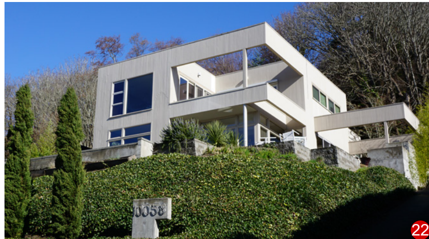
Decks; Tongue & Groove Wood; Large Windows Facing View 22
