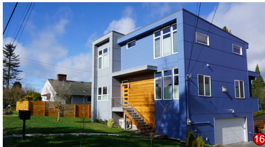
Windows Facing View; Fiber Cement Cladding; Canopy; Wood Entry
