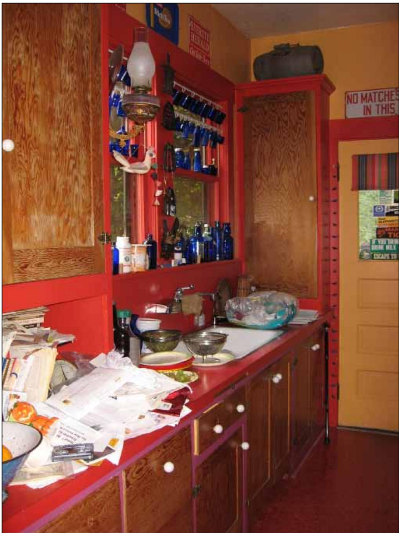
2010. View of original, wood kitchen cabinets including cooler (narrow cupboard above counter next to back door). Facing southeast. Existing countertop and vinyl floor installed in the 1970s. Source: Historic Seattle
