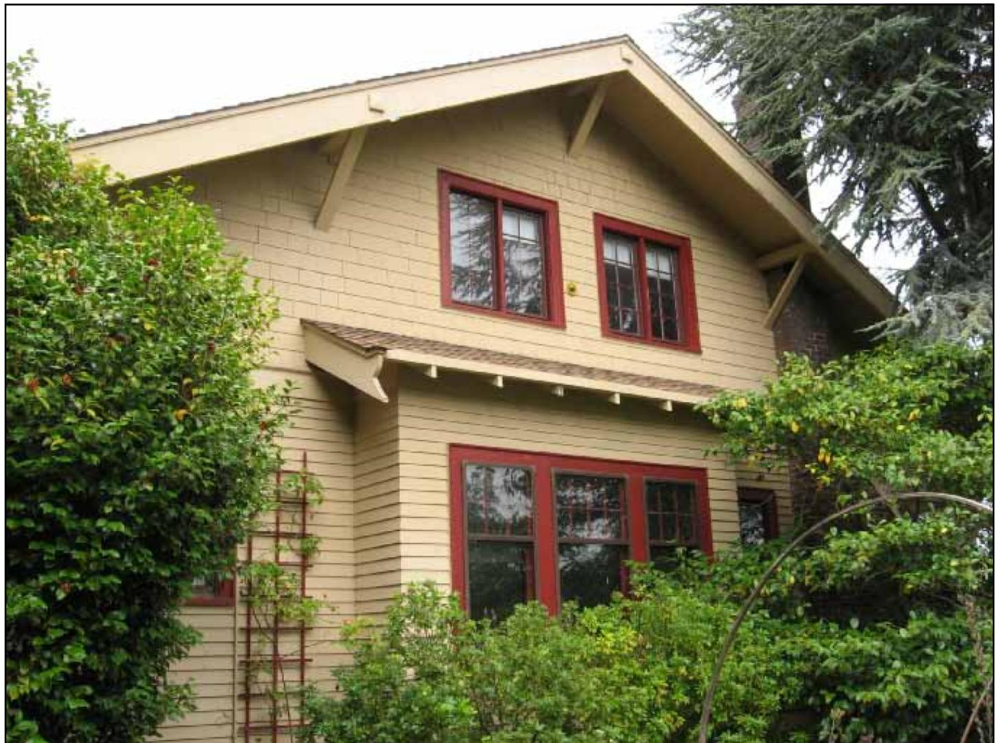
2009. View of east facade, facing northwest. Square window bay features a cluster of three, original, double-hung-wood sash windows (with contemporary storm windows). Bay has a shed roof with notched vergeboard end and rafter ends. Original casement windows provide light into the upper half-story.
