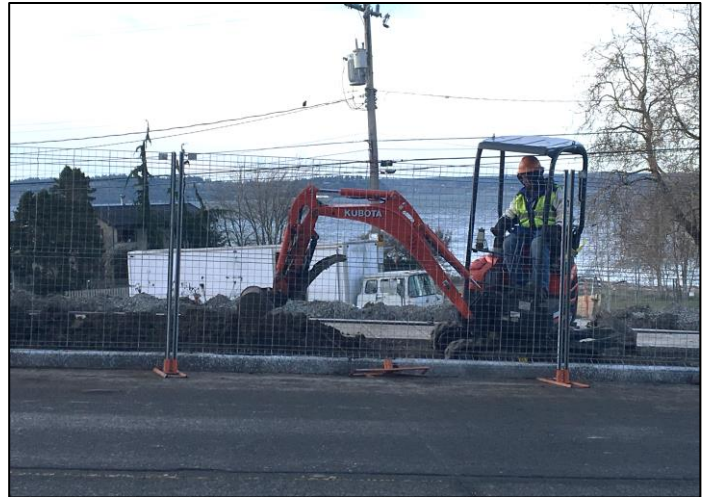
Crews prepare soil for planting on Beach Dr. S.W.
